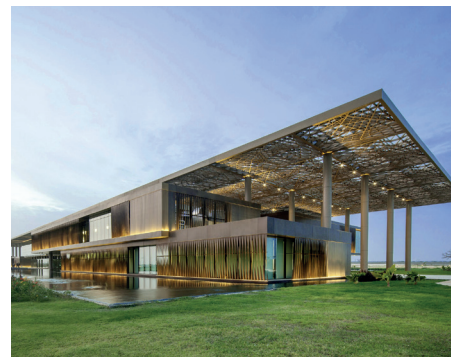
Data Center Senegal
